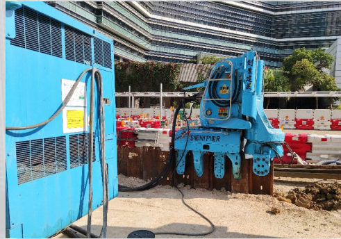
Removal of sheet-pile by silenced type Powered Mechanical Equipment (PMEs)
