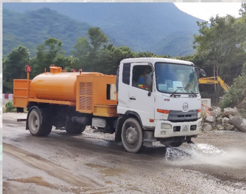
Water spraying by water truck along haul road
