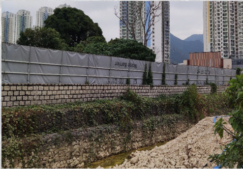
Deployment of noise barrier
