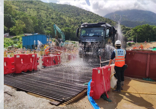
Wheel washing facility at the site exit
