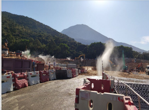
Water spraying via sprinklers at construction site for dust suppression
