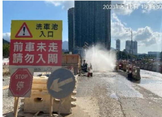
Wheel washing bay with high pressure jet
