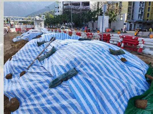
Covering excavated stockpiles by impervious sheeting
